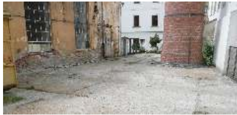
(a) Chimney location
