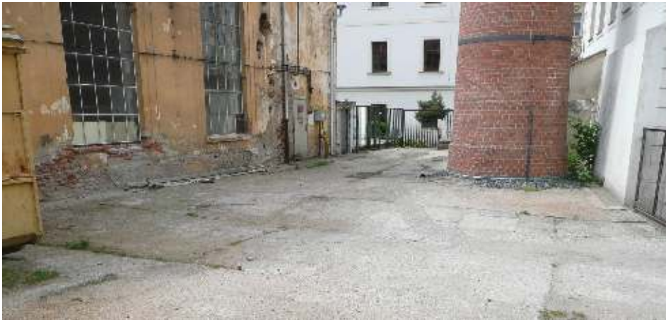
(a) View of the chimney location.
